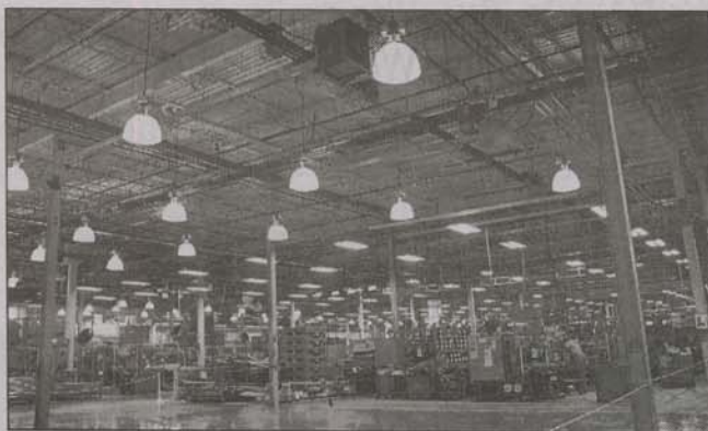
New energy-efficient lighting, whose intensity will not erode over time, has begun replacing the old bell-shaped lighting, which loses 50-percent of its intensity in the first 18 months of use.
